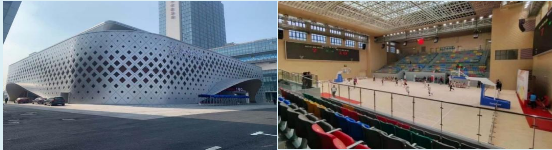
Venue of Shanghai Songjiang Stadium 38 Ledu Road, Shanghai
