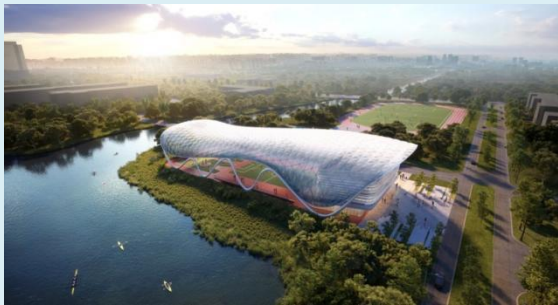
New Venue of Shanghai University of Engineering Science 333 Longteng Road, Shanghai
